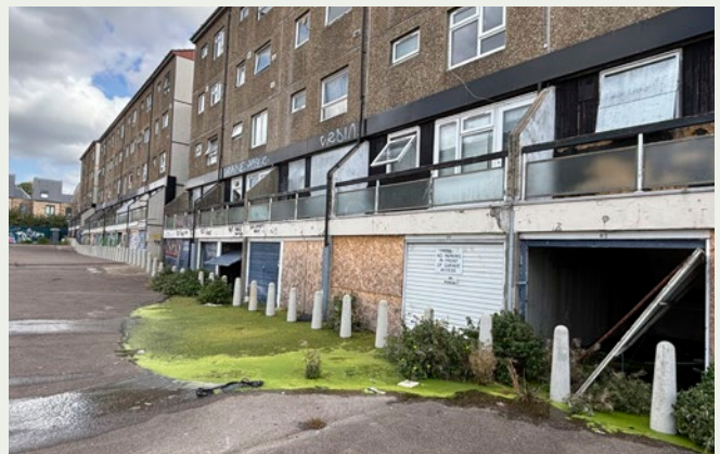
Vandalised flats at the Dollis Valley Estate
