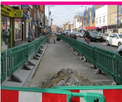
Building work is in progress to construct the pavement build-outs
