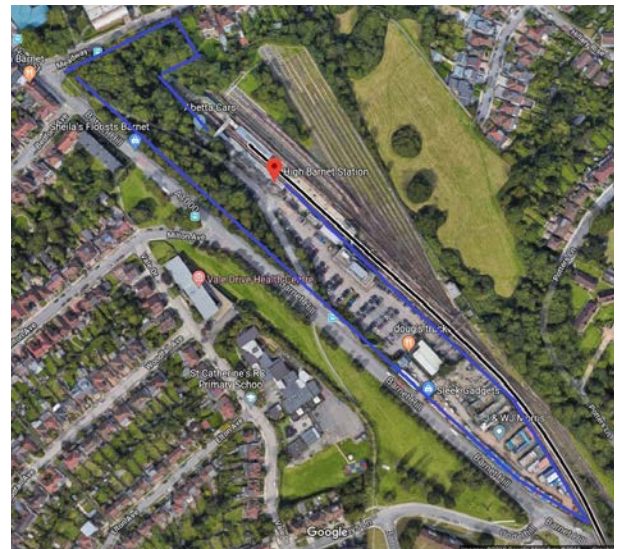
Aerial view of the proposed site of the apartments
