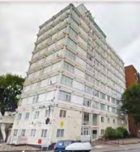
1 Station Road prior to its conversion
