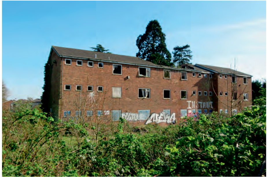
The fire-ravaged and dilapidated nurses home is to be demolished
