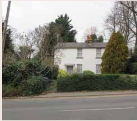
Well Cottage, at the top of Wellhouse Lane, which is the home of Whalebones tenant farmer Peter Mason, would retain sufficient land for rearing geese and poultry. Originally two cottages, dating back to around 1650, it was the home of well keepers who supplied water for the horses of the carters and drovers who stopped off in Barnet when taking hay and forage into London or when leaving with loads of horse manure and ash.
