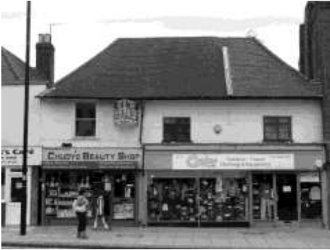
“Cover” shop before,
