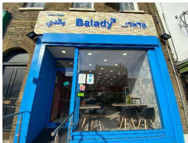
60 High Street: shopfront built without permission
